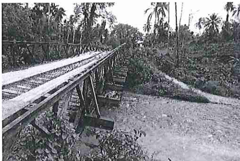
Example of damaged bridges along the Northern Road (Kwai & Sulagwalu Bridge)
